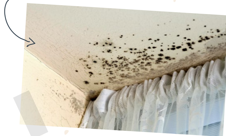
Example of mould in a student house
